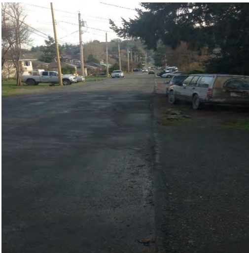
Figure 6- Pear St. is very narrow, there is no pedestrian or cycling infrastructure.
